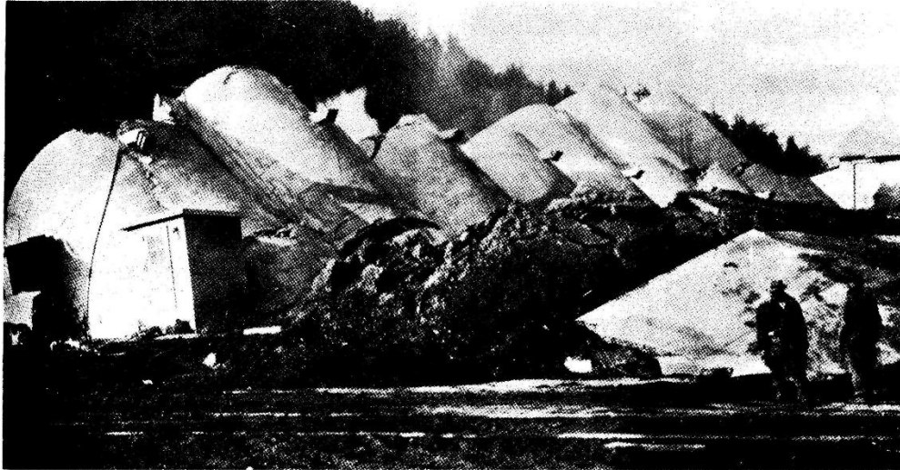
Bearing capacity failure of a silo foundation. (From Tschebotarioff, 1951.)
