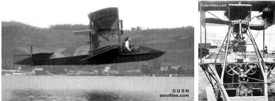
**Figure 1.14:** Aircraft autopilot system. The 1912 Curtiss (left) used an autopilot to stabilize the pitch of the aircraft. The Sperry Autopilot (right) contained a set of four gyros coupled to a set of air valves that controlled the wing surfaces. The Sperry Autopilot was able to correct for errors in roll, pitch and yaw [Hug93].
