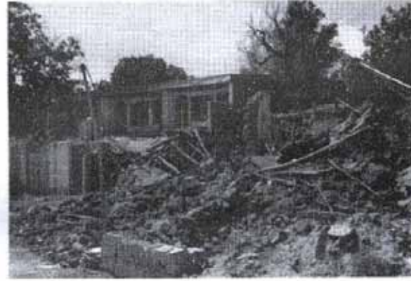
Fig. 10: Collapsed non-engineered buildings beside engineered ones
