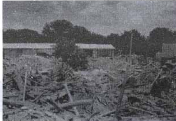
Fig. 8: Complete failure of adobe buildings in Changureh
